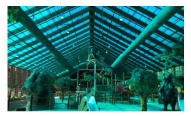
Five wall increases the R Value over traditional twin wall polycarbonate. The material is extruded with three inner layers of polycarbonate to create more air pockets, thus increasing the R Value. This makes Macrolux® Five Wall an ideal covering for all greenhouse applications where heat saving is a concern. It is also ideal for industrial and residential building such as:
